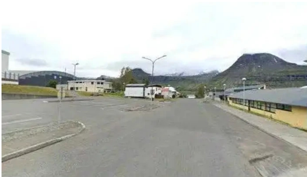
Íþrottamidstod reyðarfjardar street view 360deg
