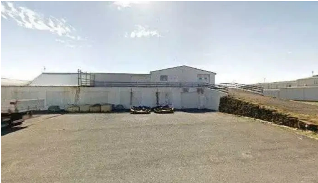
Slokkvistod grindavik street view 360deg
