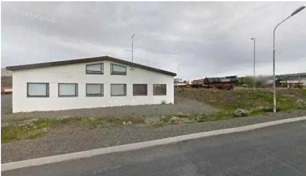
Slokkvilid borgarbyggðar street view 360deg
