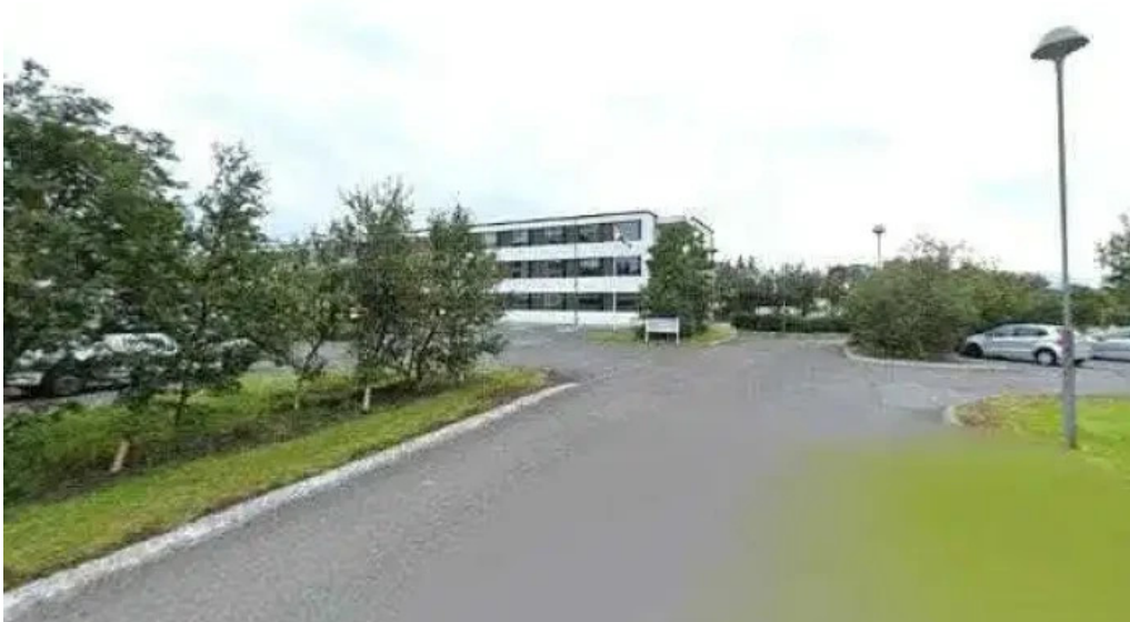
Landspítali grensas street view 360
