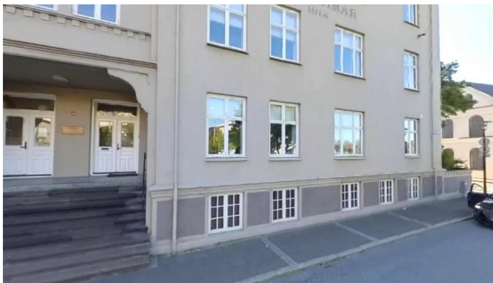
Umbodsmadur althingis street view 360deg
